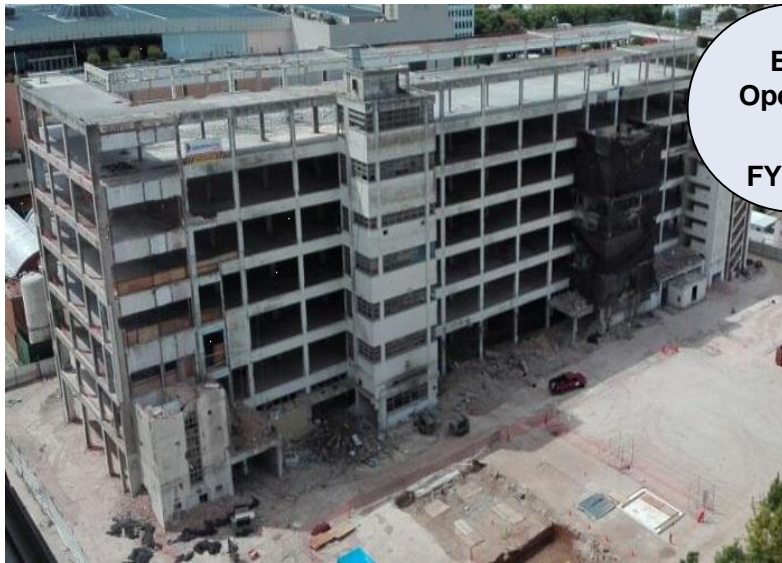
Construction Works (Current Picture)
