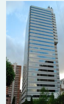
Intercontinental (A) – 3 floors remaining
