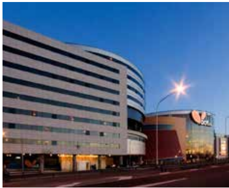
DOT BUILDING Buenos Aires
